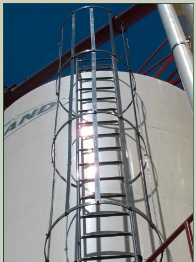
The safety hoop ladder offers a greater degree of safety than the traditional types.
